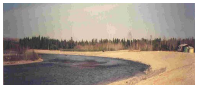
Remediated Cave In Site after spring ice flow
